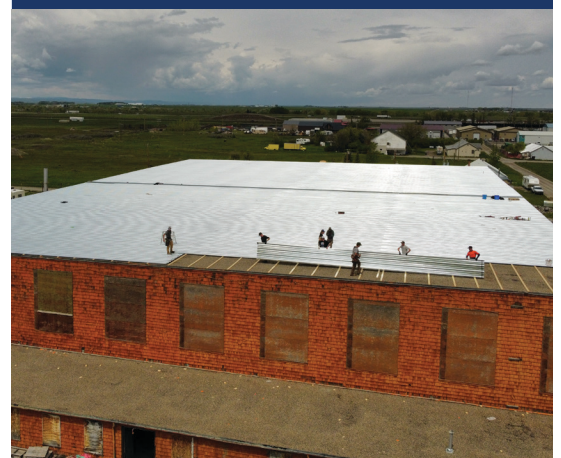
Pictured is a roof in Galvanized.
